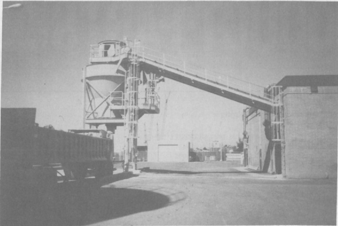
Overall view of sludge silo with ROPLEX at outlet.
